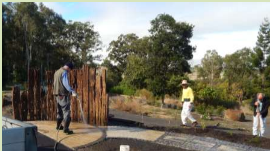
Will, John and Don putting finished touches to old fence post wall and mosaic pathway. We are now looking forward to the growth of the plants in this area
